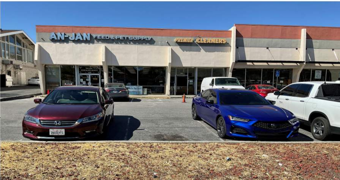
Due to the grade changes from the street to the business entrances, Protrk relocated the ADA parking stalls, so the ADA compliant access aisle could perform double duty by also serving as the path of travel to the city sidewalk, avoiding costly ramping and railings.
