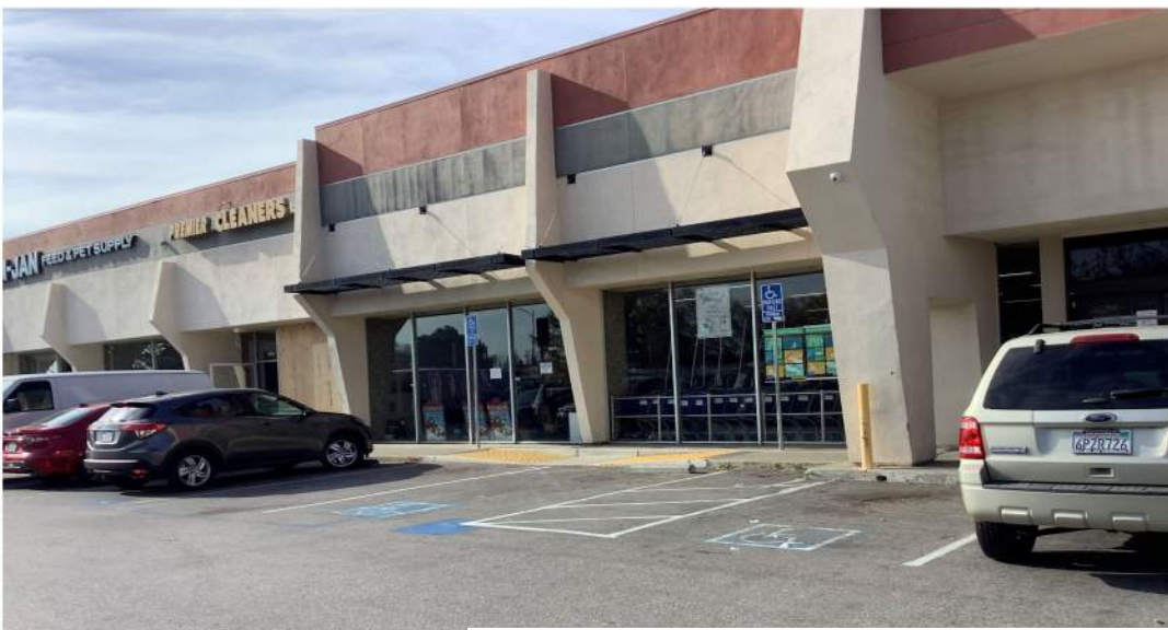
This older development was flagged by a CASp report with numerous barriers to be remediated: the store front sidewalk cross slope was non compliant, several unsuccessful efforts had been made to correct the ADA parking layout, and there was no accessible route to the public sidewalk.
