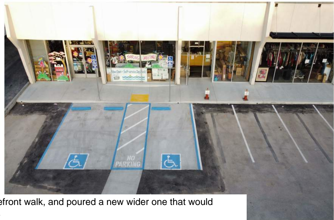
This older development was flagged by a CASp report with numerous barriers to be remediated: the store front sidewalk cross slope was non compliant, several unsuccessful efforts had been made to correct the ADA parking layout, and there was no accessible route to the public sidewalk.
